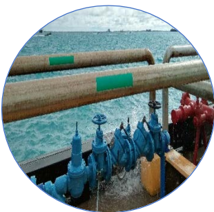
Figure 4. Sub Site service line #2 found at the wharf
