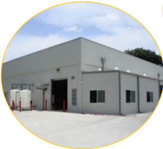
Figure 2. Main WTP at Cantonment
